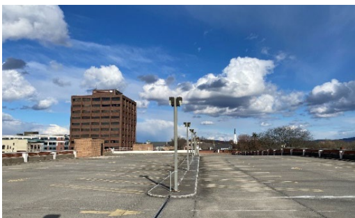
The top floor of the Walnut Street Garage
