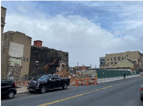
Project I: Boyd Theater Demolition Site
